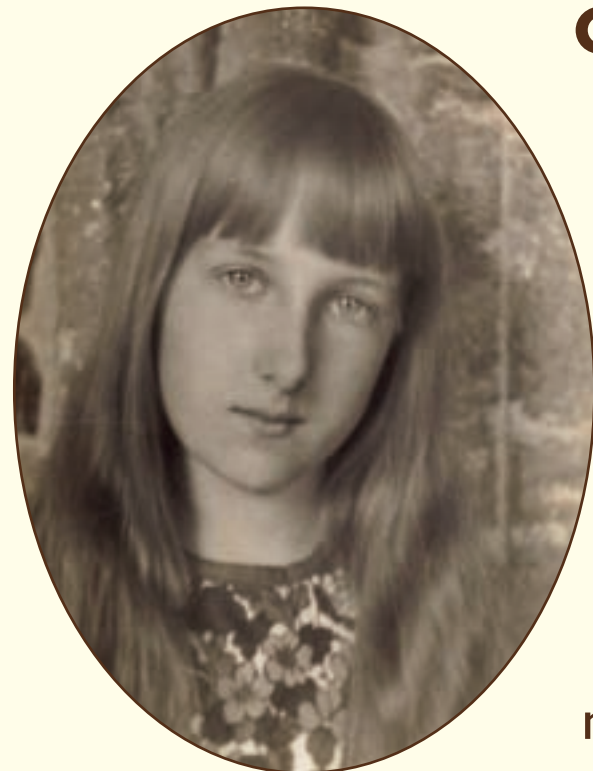
Imogen in the porch of Thaxted Church, 1919.
